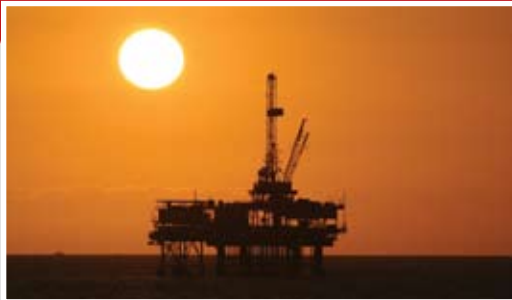
Oil and gas pipelines Offshore platforms
