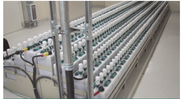
FNC® stationary battery system
